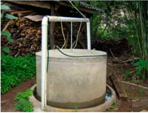
The floating biogas tank GEI installed for Changshui peasants
