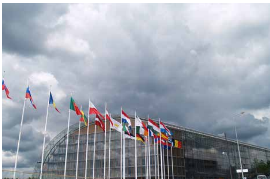
European Investment Bank building in Luxembourg, photo Re:Common/2009
